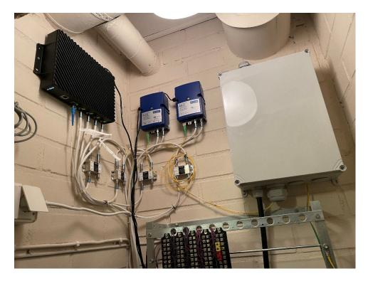
By extending its fiber network to each building and repurposing the existing coaxial network, previously used for cable-TV, PSSV could provide a fiber-like broadband performance to individual tenants residing in the MDU.
